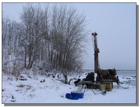
b. Drilling at Test Boring AP-622 with helicopter portable drill rig. December, 2006.
