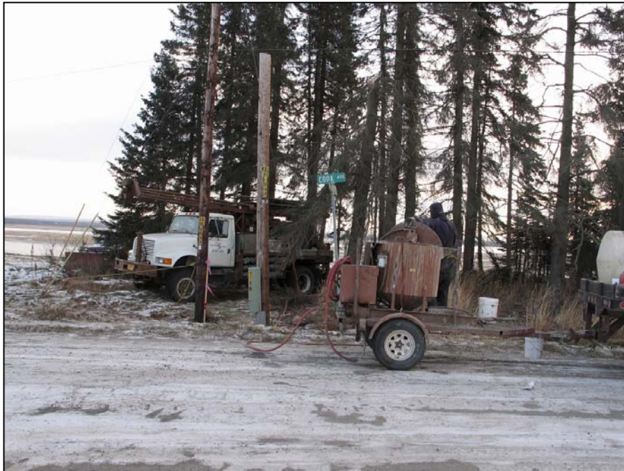
b. Grouting at Group 2 borings. November, 2006.
