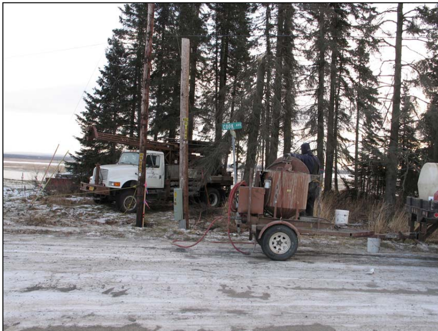
b. Grouting at Group 2 borings. November, 2006.
