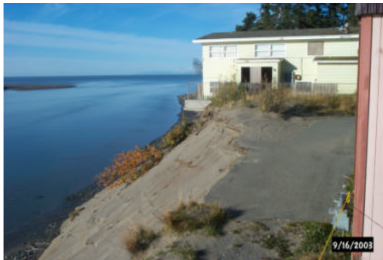
Undercutting of existing structure by receding bluff.
