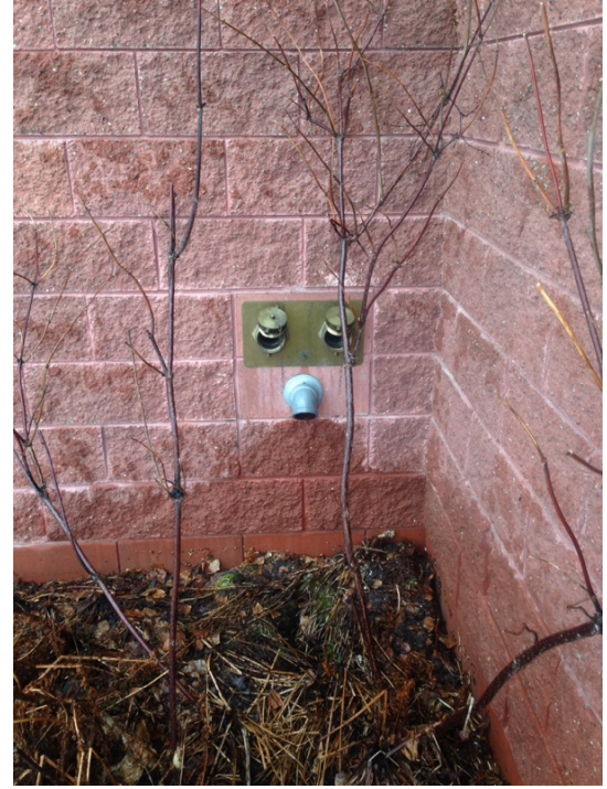
Fire department connection inspection
