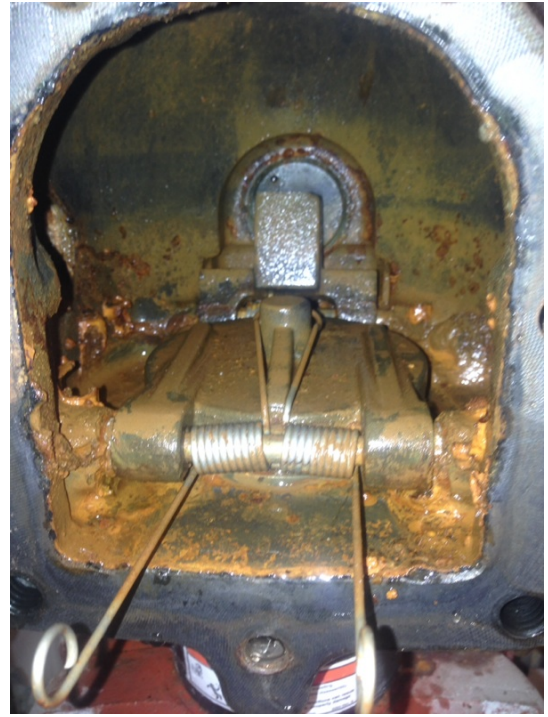
Internal Dry valve inspection
