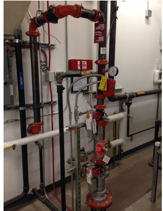
Riser tagged and in the proper state prior to leaving
