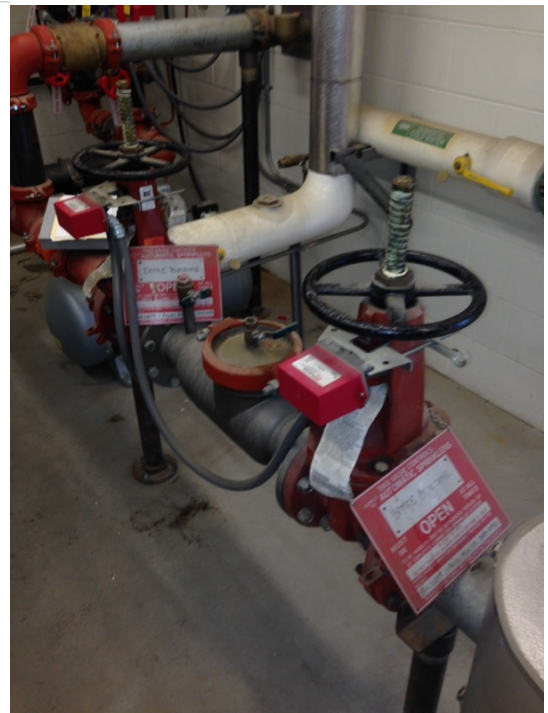
Internal Dry valve inspection
