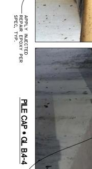
APPLY INJECTED -REPAIR EPOXY PER SPEC, TYP.
