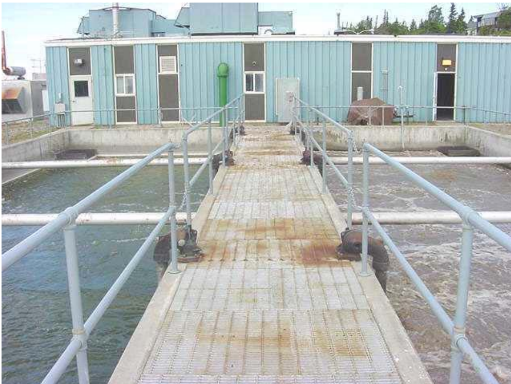
PHOTO 5-5 Aeration Basin Catwalk
