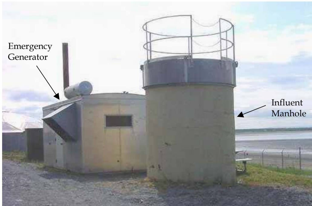
PHOTO 5-1 City of Kenai WWTF Influent Manhole
