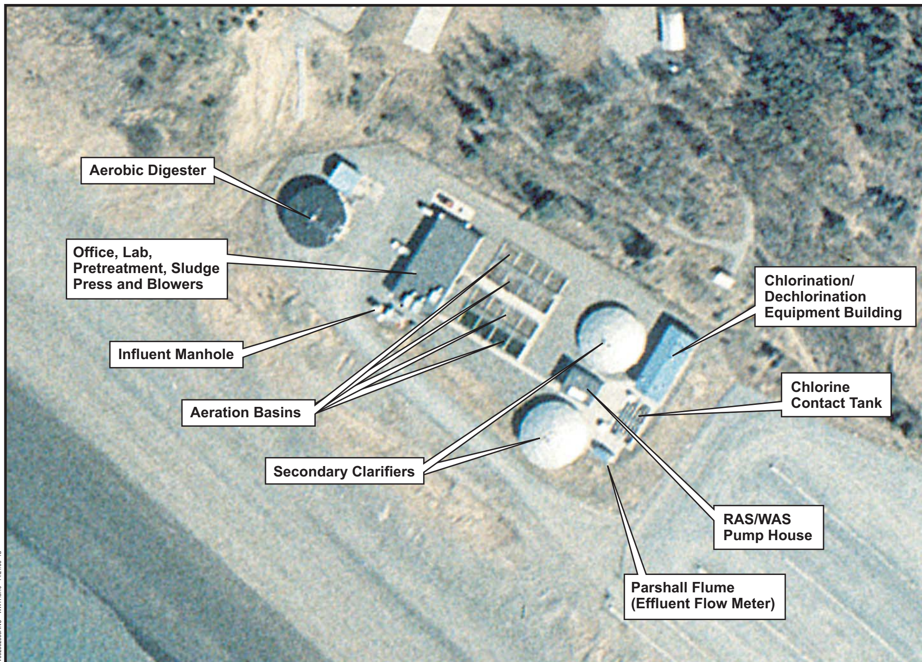
Figure 2-5 Waste Water Treatment Facility Kenai, Alaska
