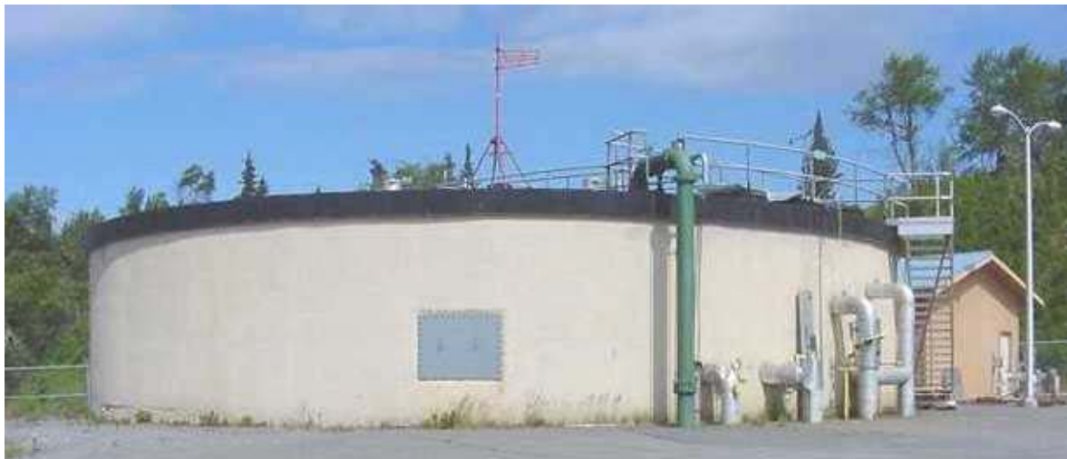
PHOTO 5-14 City of Kenai WWTF Aerobic Digester
