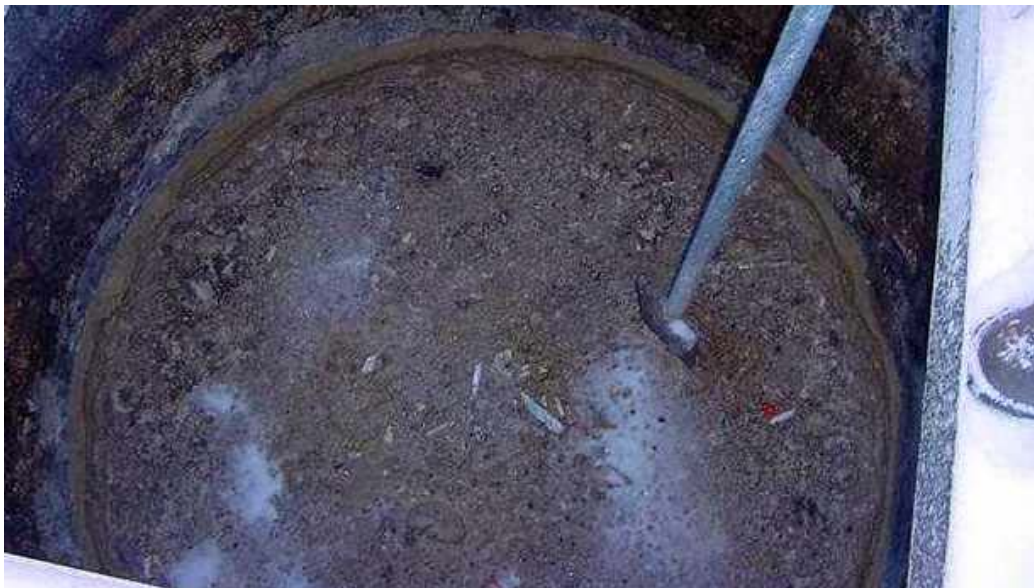
PHOTO 5-2 City of Kenai WWTF Influent Manhole Grease
