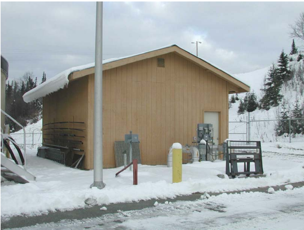
Septage Receiving Area
