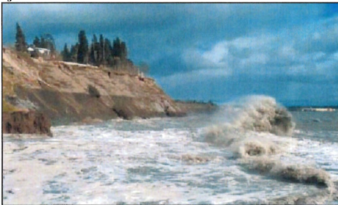
Figure 7. Storm Event at Kenai Bluffs
