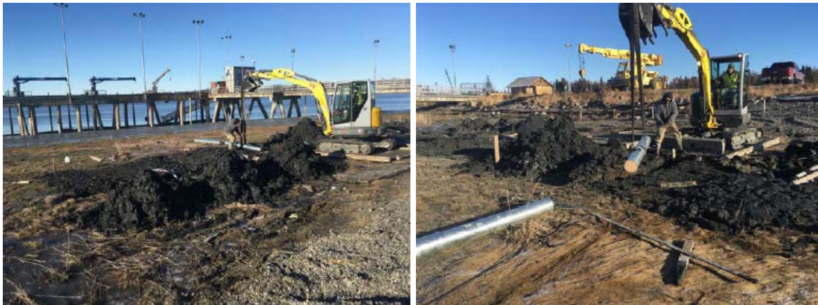
Cathodic Protection Anodes being installed
