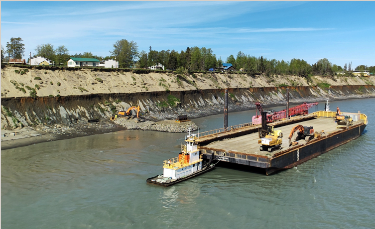
Kenai Bluff Stabilization Project underway!
