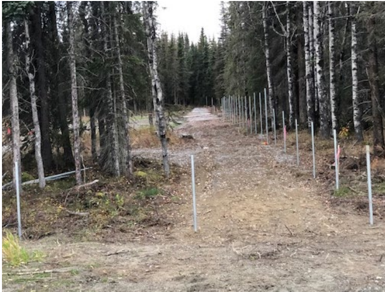
Fireweed Fence placing posts
