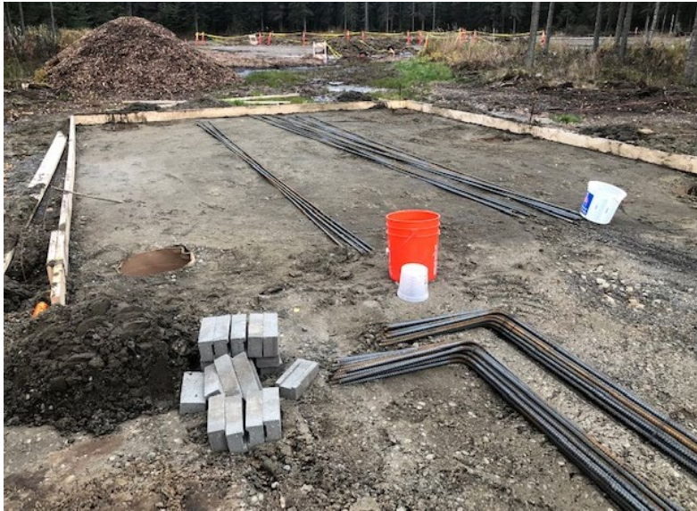
Pavilion Pad prepping for concrete
