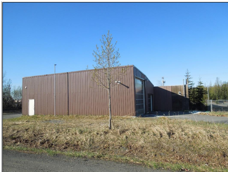
South view of property from Cohoe Avenue
