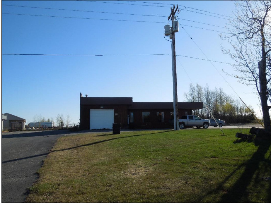
Northeast view of property from Kenai Spur Highway
