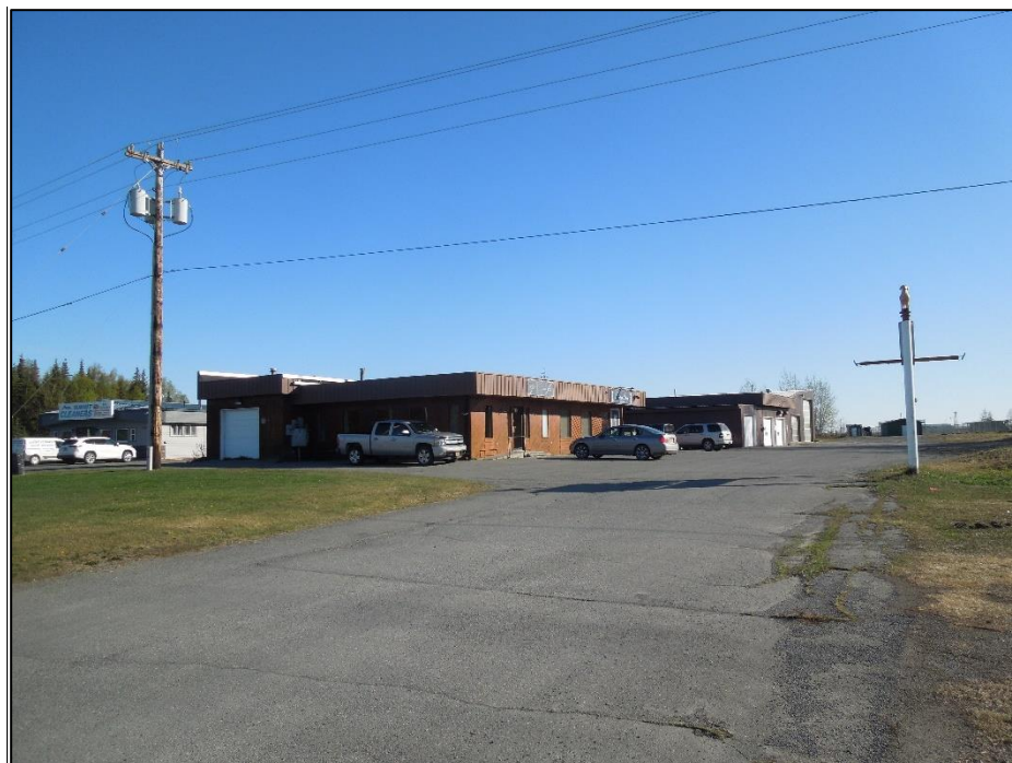
North view of property from Kenai Spur Highway
